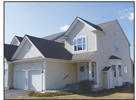
40 Bagnell Drive, Pembroke
